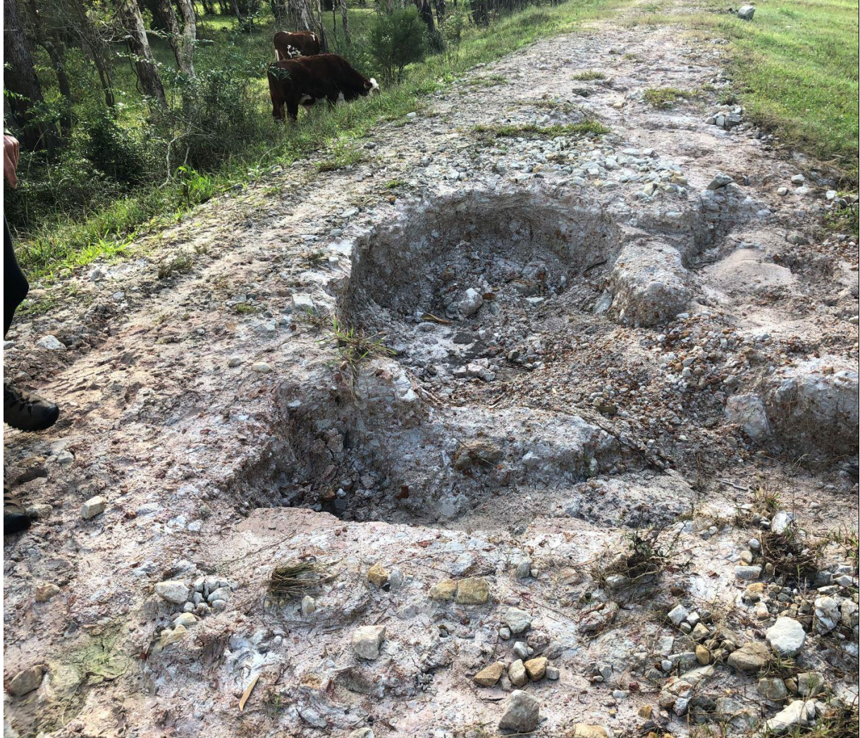
Image 4 - One of the several minor erosion \ scours as a result of levee overtopping.
