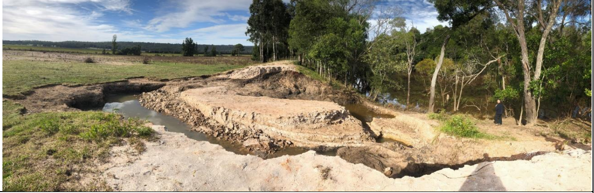
Image 4 - One of the several minor erosion \ scours as a result of levee overtopping.
